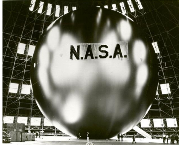
Figure 3. NASA passive communications satellite Echo II: A 41-meter diameter/36,000 cubic meter Energy Bag volume equivalent ( courtesy NASA ).
